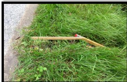
The verge starts to drop off after only 10cm at this point, and sharply drops at 30cm.
