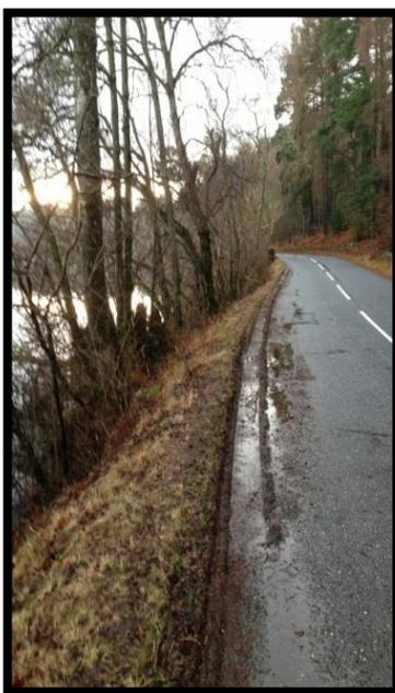
On this stretch of road immediately after a blind corner, the asphalt is too narrow at points for two lorries to pass, with tyres already often using the narrow wetlands verge.
